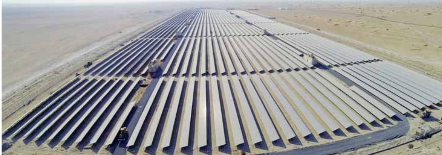
Credit: First Solar
