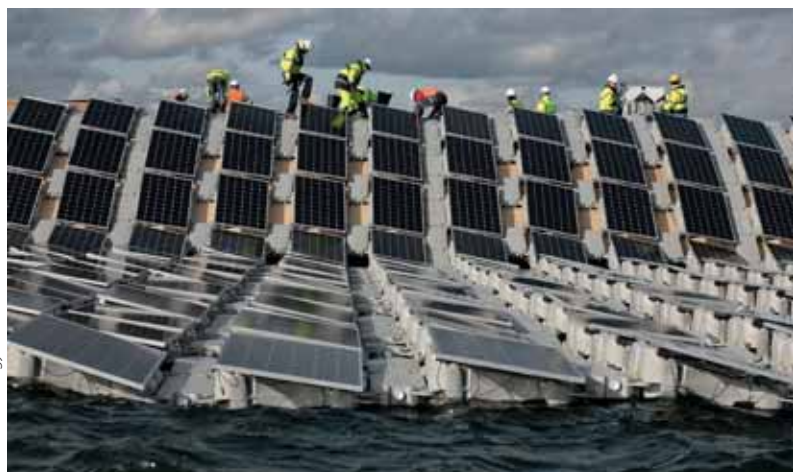
Credit OST Energy
