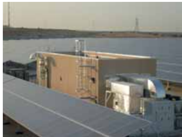
Phoenix Solar's Kapsarc project revealed the importance of humidity in the choice of module cleaning regimes.
