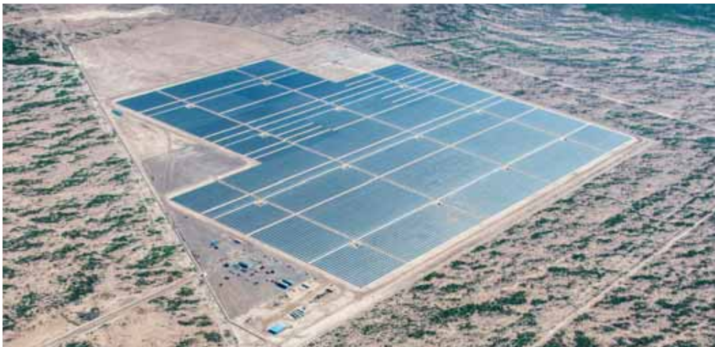
Credit: First Solar
