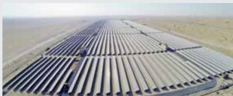
Credit: First Solar
